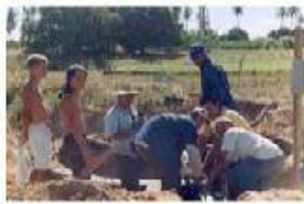
The brethren pitching in to get the plantation irrigation up and going
