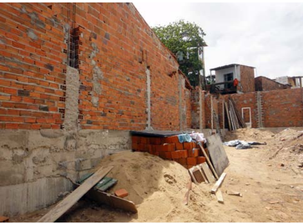
Building the walls of the new hall (see plan previous page)
