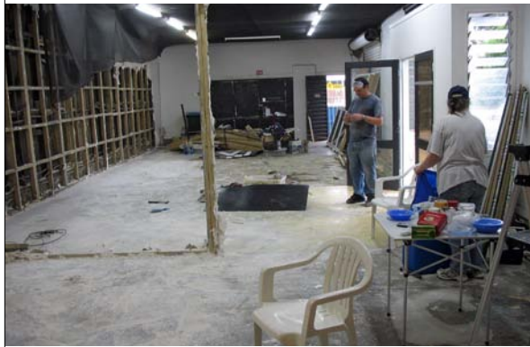
Renovating the Auckland hall
