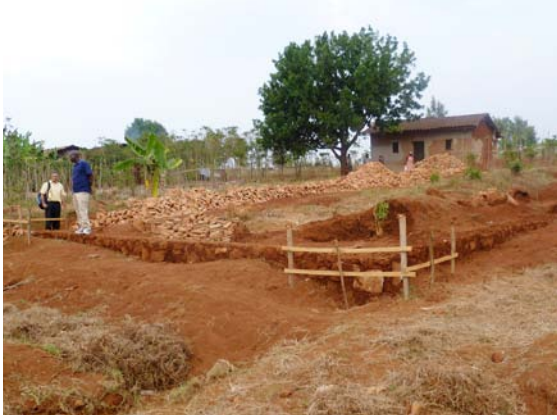
Preparing to build the hall at Mutaho
