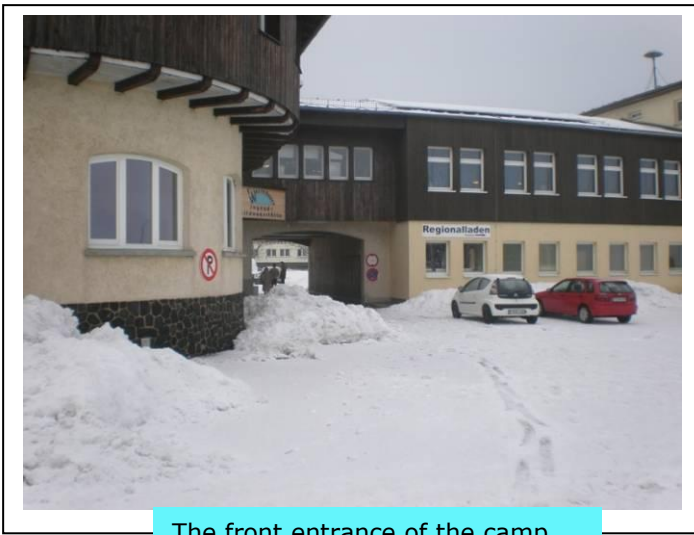
The front entrance of the camp
