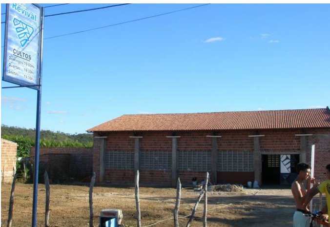
GADELHA: The new Hall built with help from Australia
